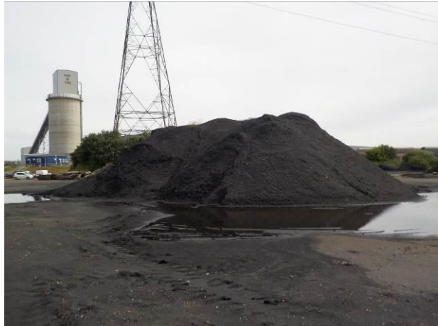
(8) Looking east. Coal storage in the southern area of the site.
