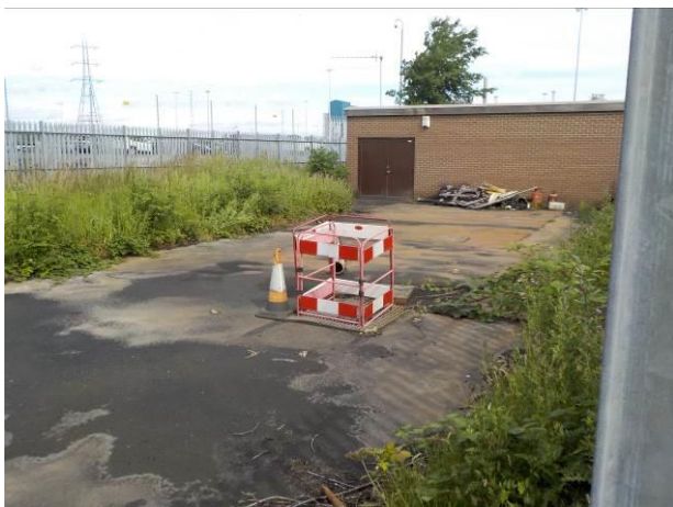
(21) Sewage pumping station to the west of the site.
