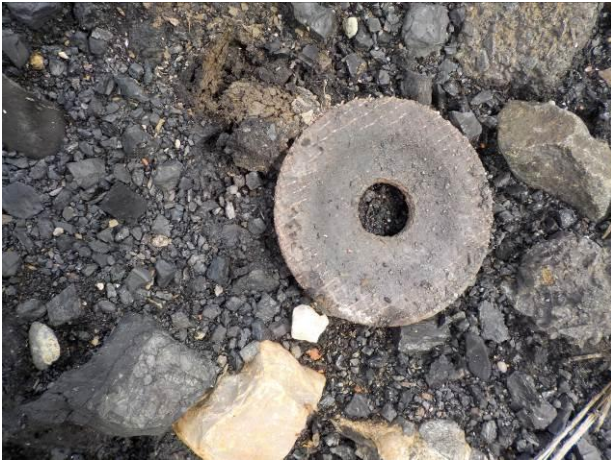
(13) Suspected asbestos gasket.
