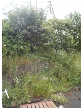
(26) Eastern boundary of the site, potentially unstable bank side.
