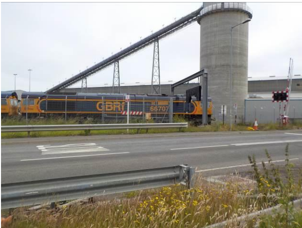
(27) Road and railway line off-site to the north.
