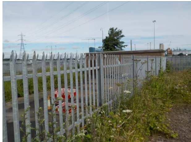
(20) Sewage pumping station to the west of the site.
