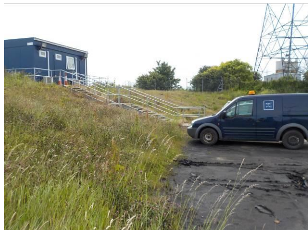
(24) Slope on the northern site boundary
